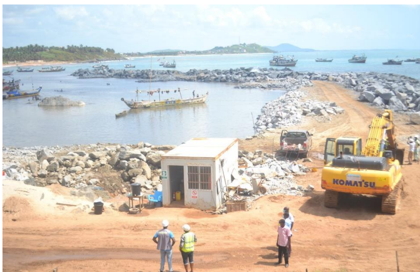
Figure 13: A picture showing the jetty being constructed for the Mumford community.
