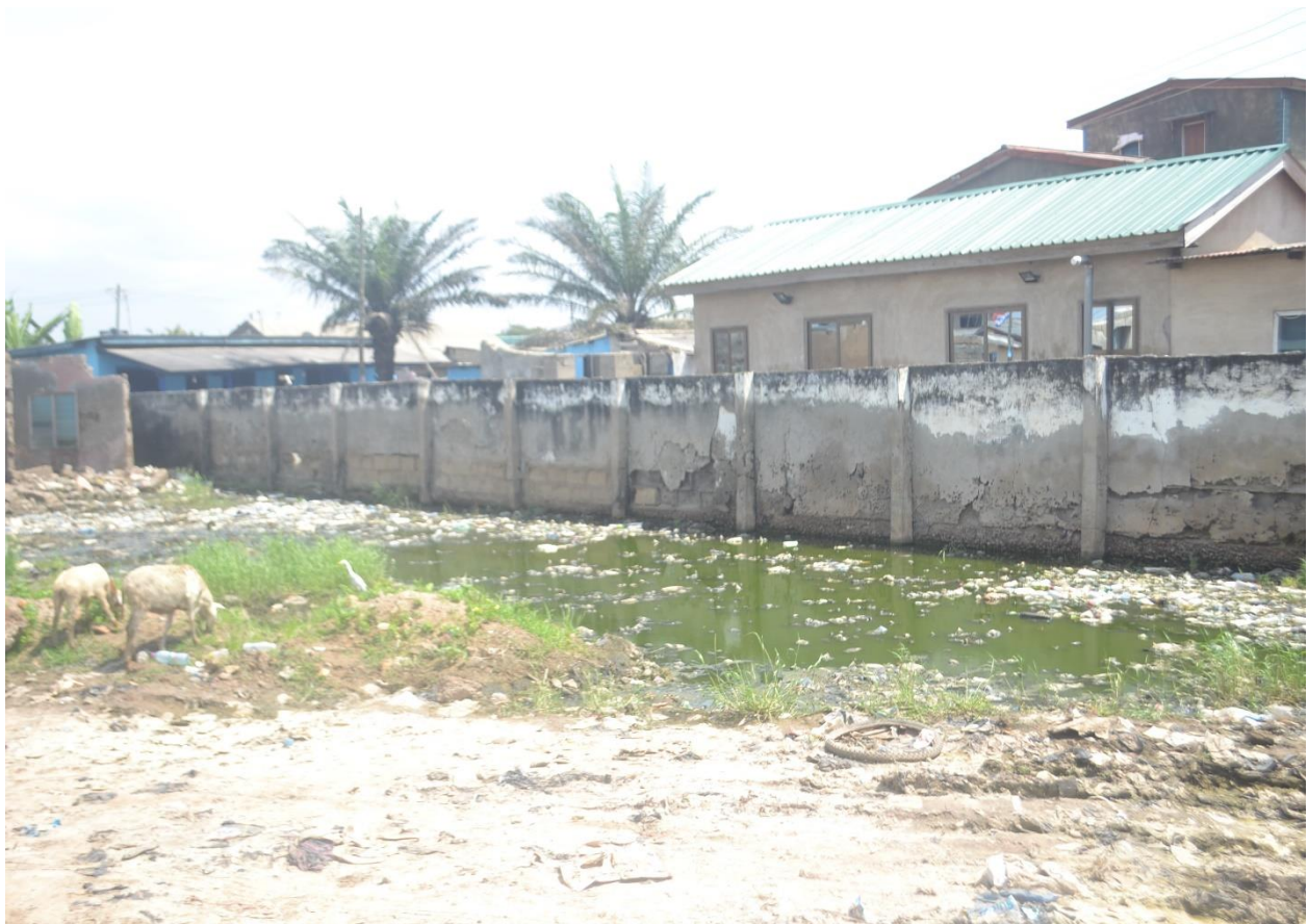
Figure 5: A picture showing some flooded areas in Opetekwei.
