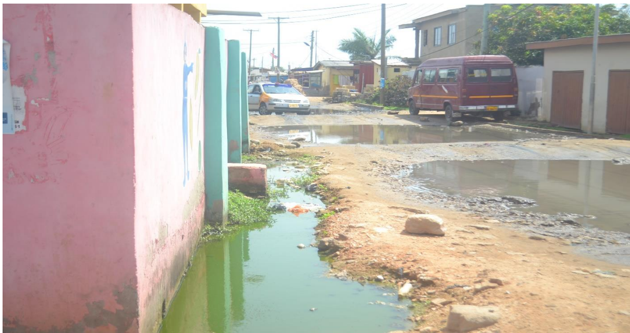
Figure 4: A picture showing house built on drainage systems.
